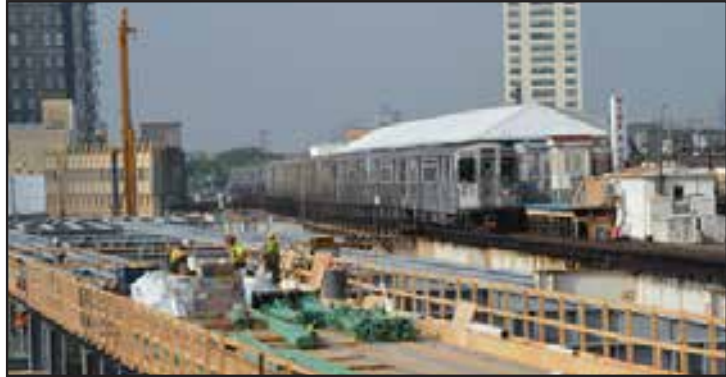
Approximately 2,200 feet of elevated tracks, signals and supporting infrastructure are being relocated as part of the Wilson Rehabilitation.
