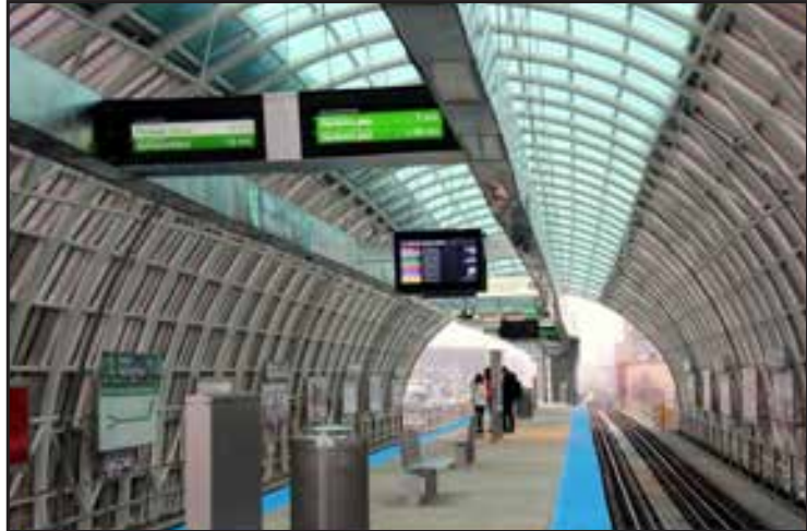
Located just two blocks from the McCormick Place, the new Cermak-McCormick Green Line station features a fully enclosed boarding platform to protect riders from the elements.
